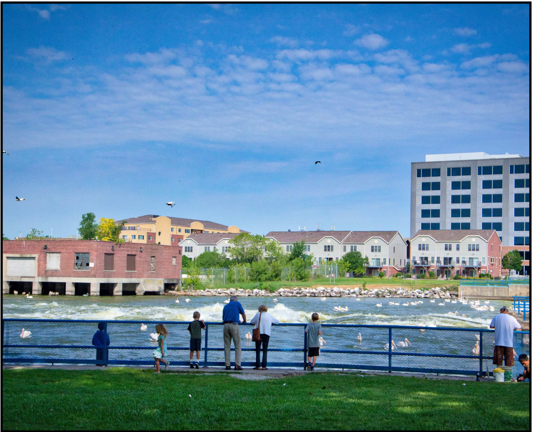
(Above) People checking out the pelicans below the dam. A couple of gates are open and the water is surging downstream. (Top Right) Pelicans looking for a meal below the dam. (Bottom Right) Wide angle view taken from the Racine Street Bridge, upstream of the dam.
